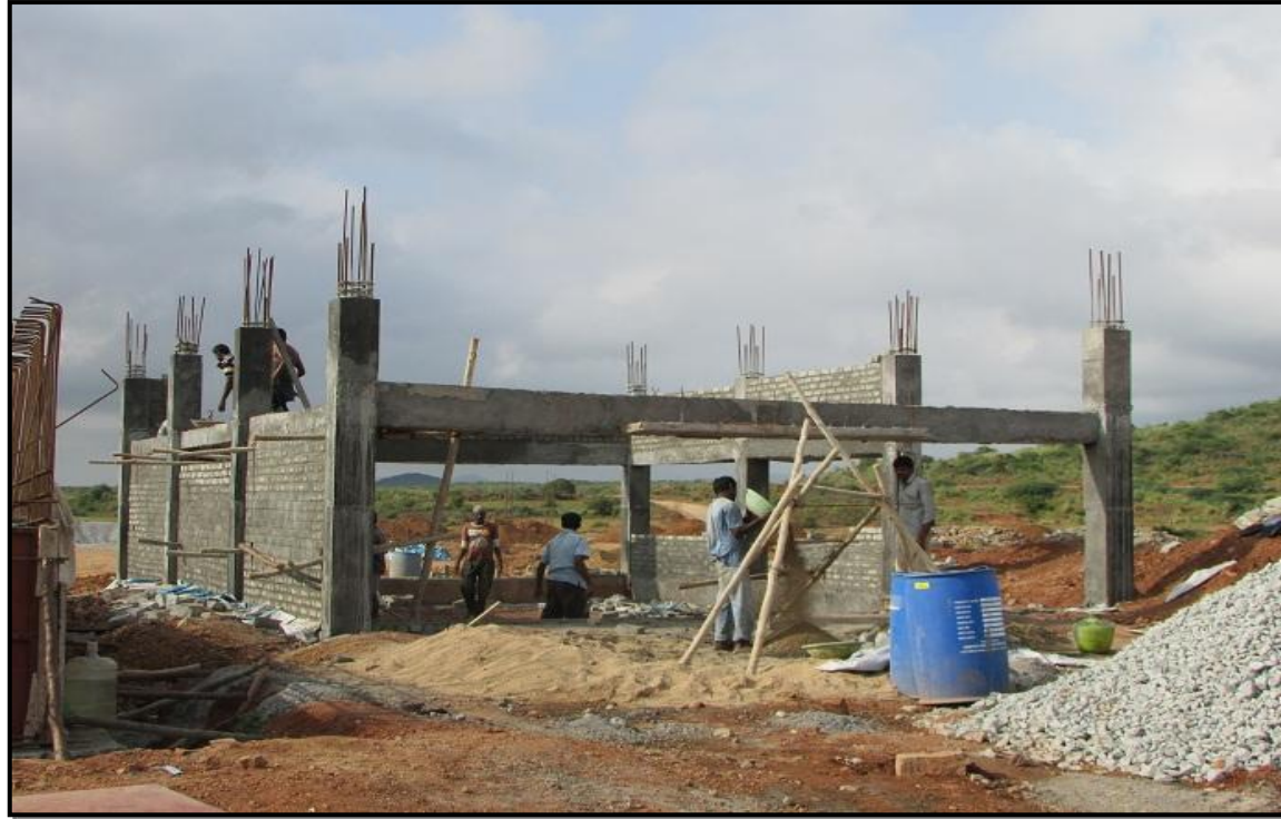
FIRE FIGHTING PUMP HOUSE BRICK WORK IN PROGRESS
