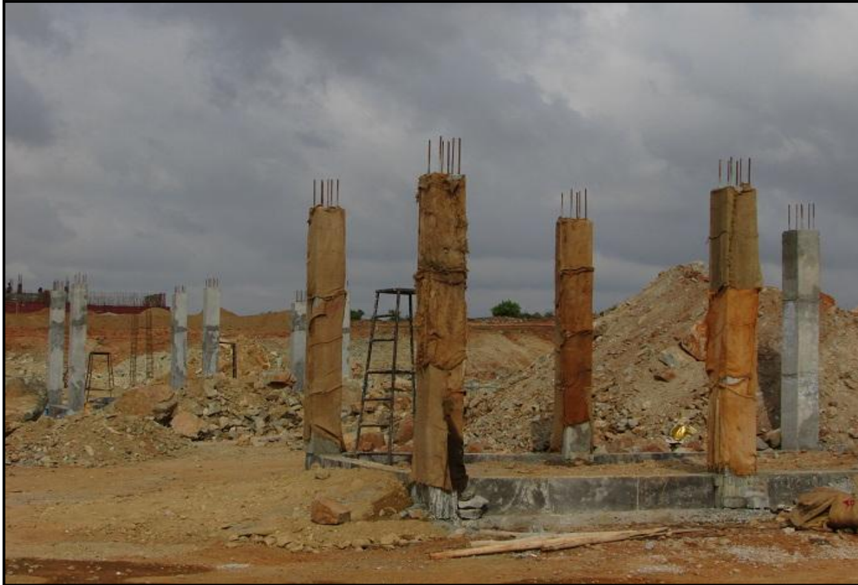
SWITCHYARD PANEL ROOM WORK IN PROGRESS
