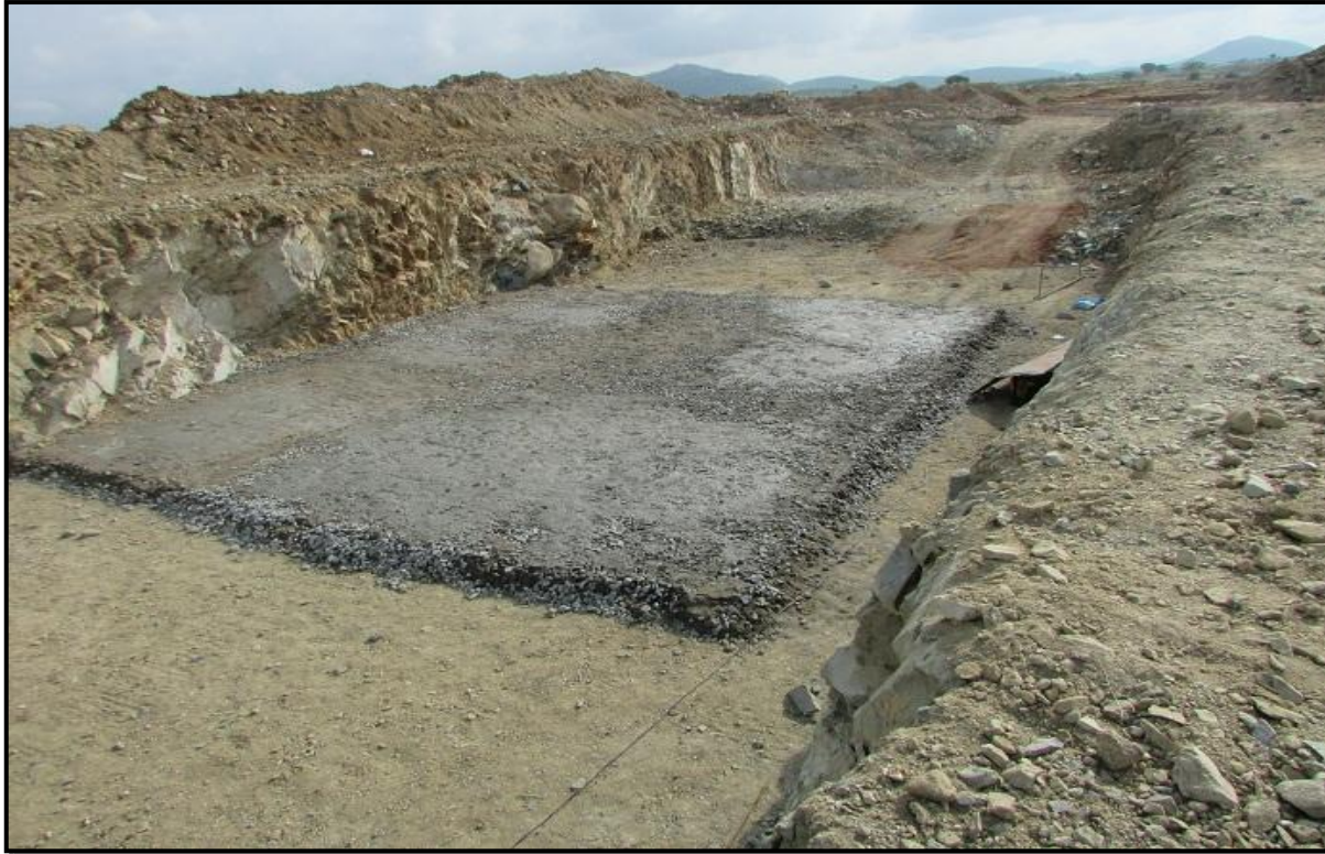
TRANSFORMER FOUNDATION WORK IN PROGRESS
