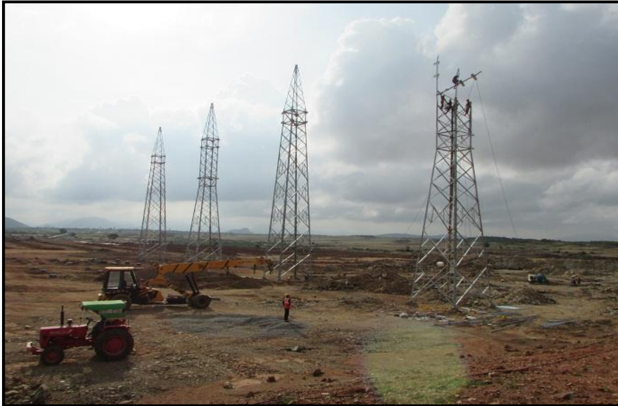
LATTICE STRUCTURES ERECTION WORK IN PROGRESS
