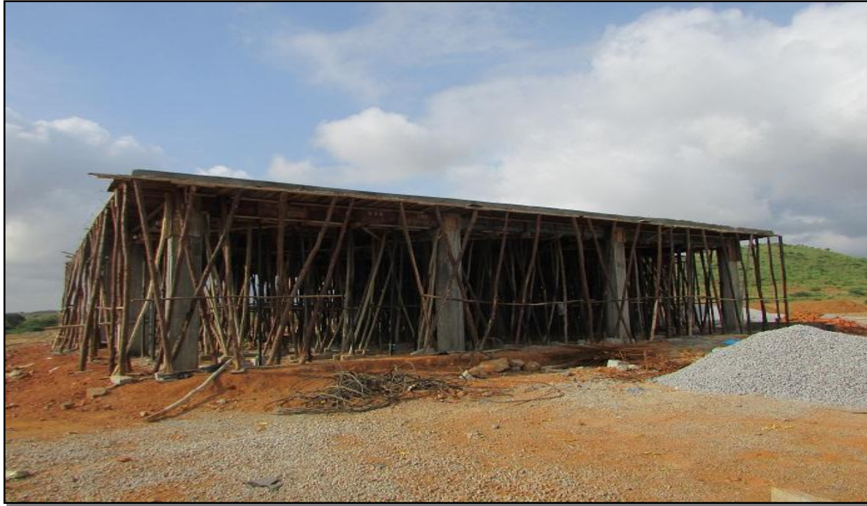
CONTROL ROOM SLAB CASTED
