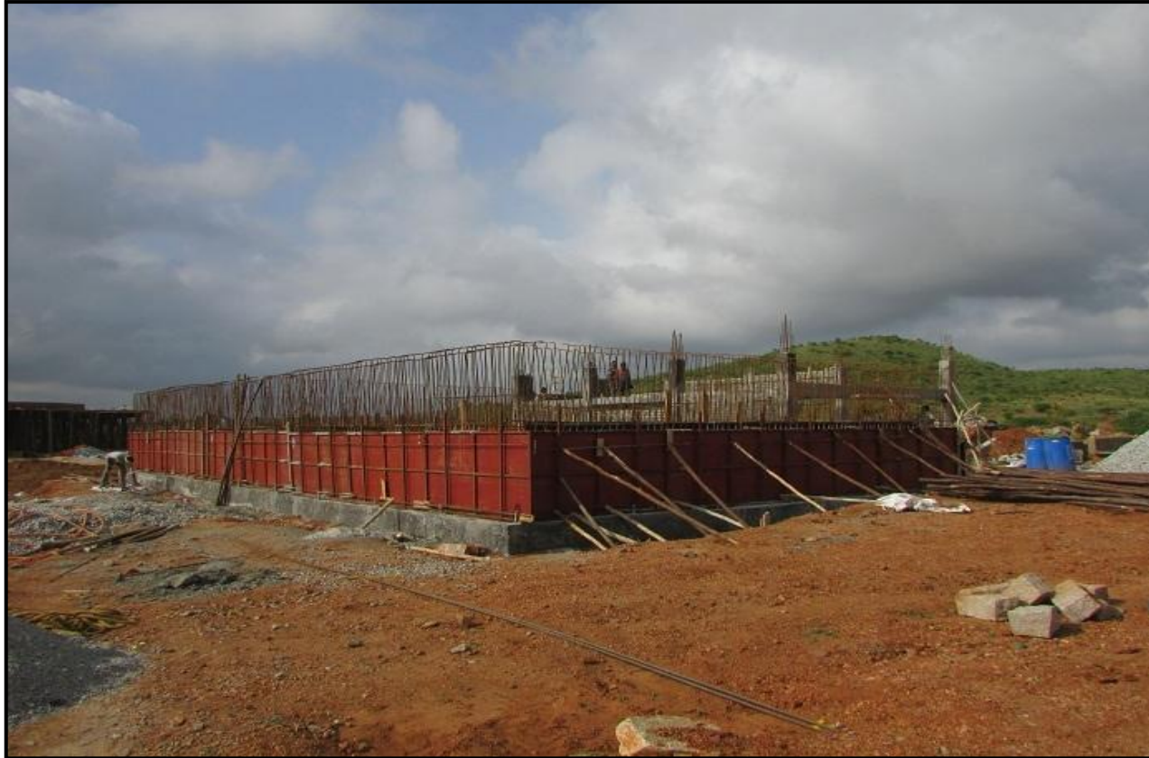
FIRE FIGHTINH WATER TANK WORK IN PROGRESS
