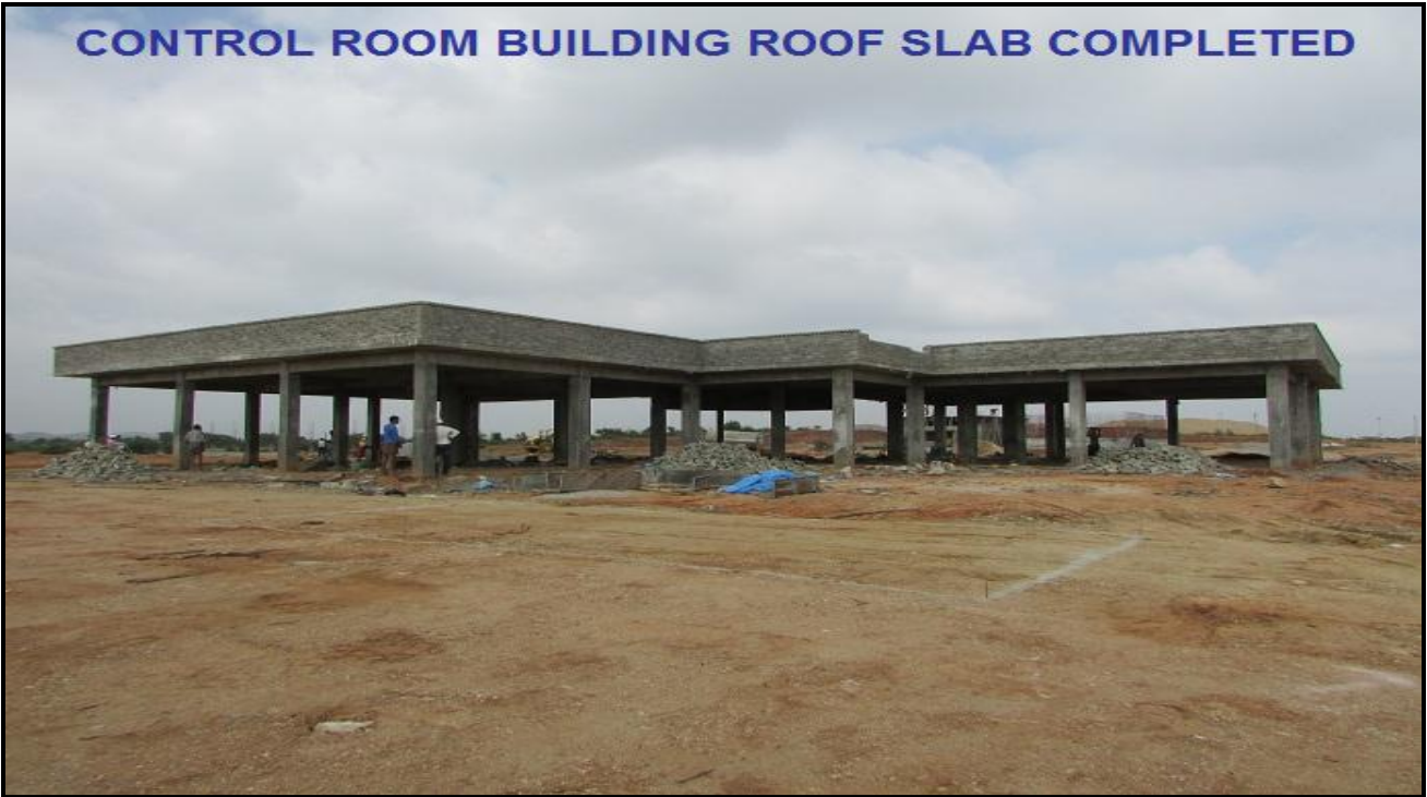
CONTROL ROOM SLAB CASTED
