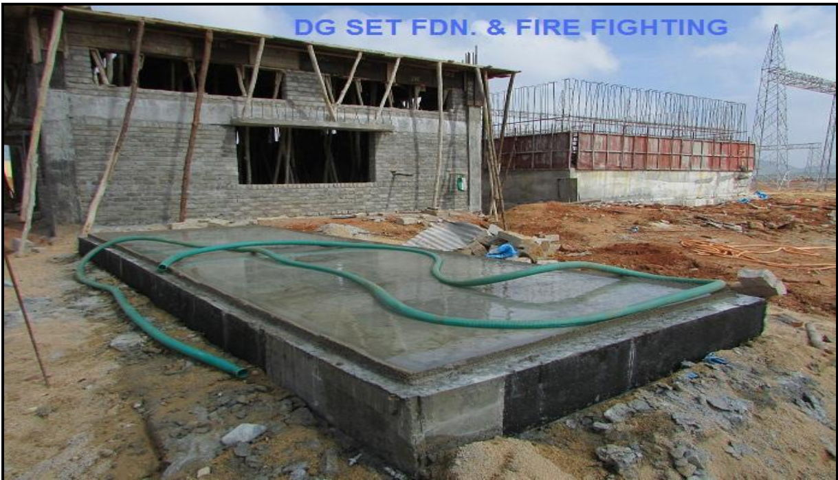
DG SET FOUNDATION & FIRE FIGHTING PUMP HOUSE WORKS IN PROGRESS
