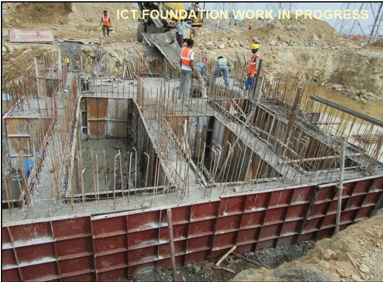
ICT-I FOUNDATION WORK IN PROGRESS
