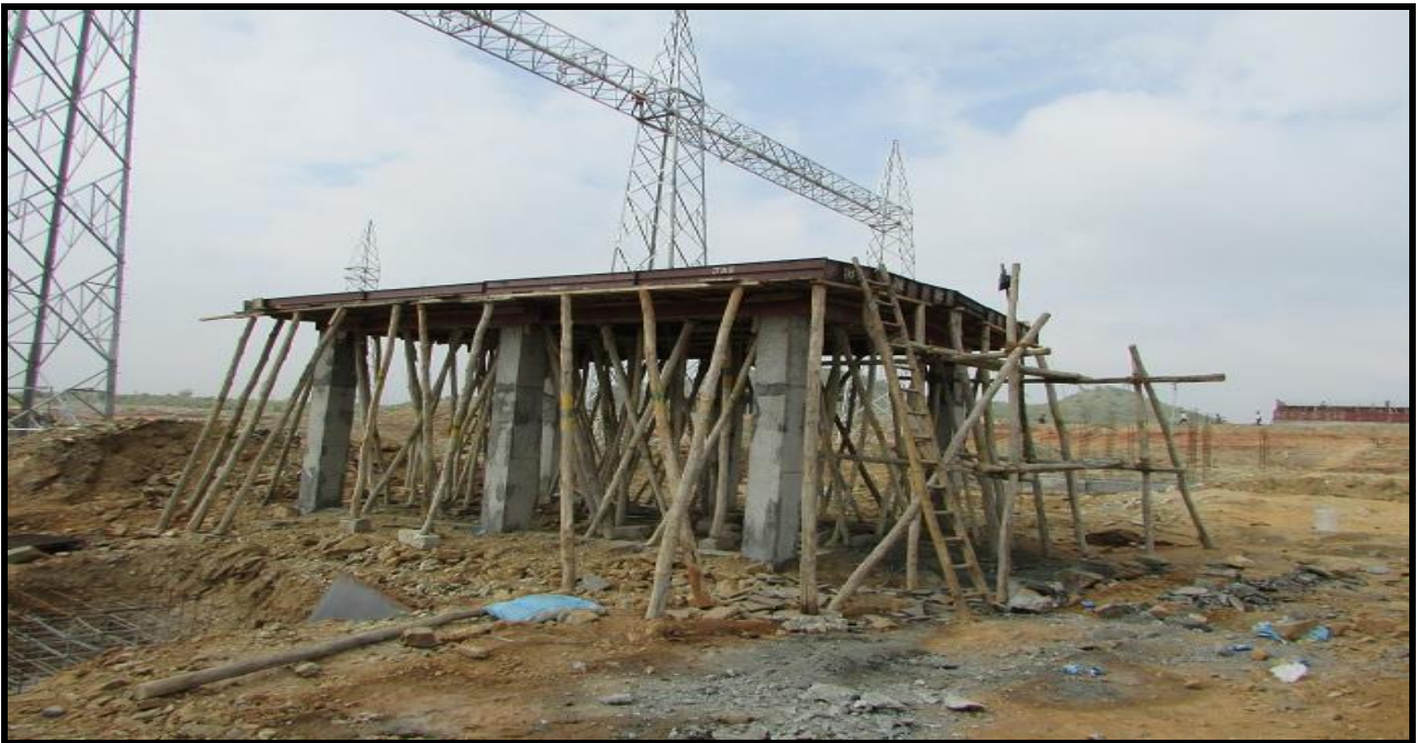
SWITCHYARD PANEL ROOM ROOF SLAB COMPLETED
