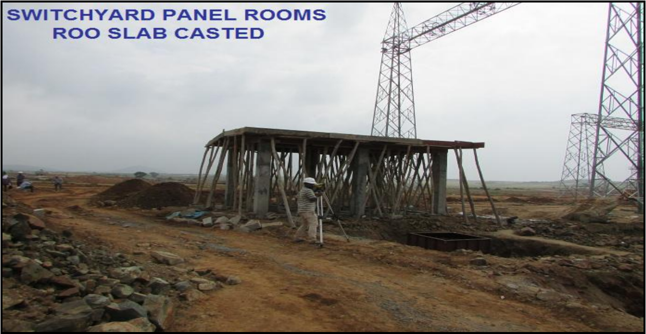
SWITCHYARD PANEL ROOM ROOF SLAB COMPLETED
