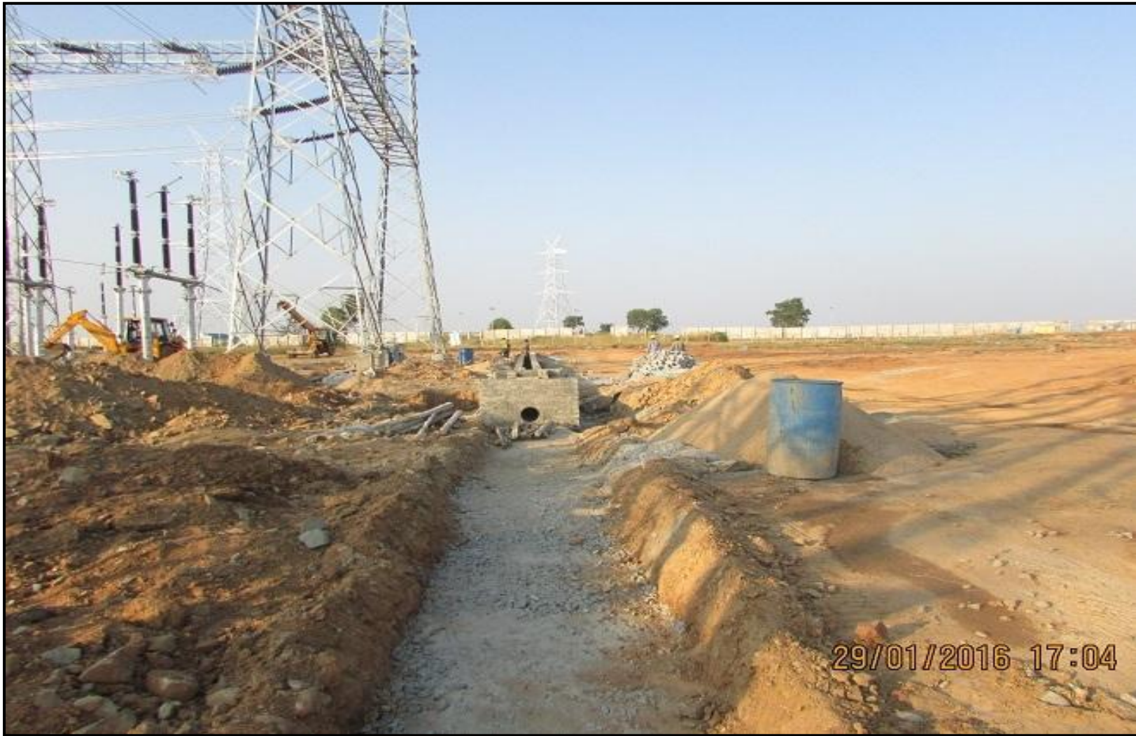
SWITCH YARDS DRAINS WORKS IN PROGRESS AT NP KUNTA 400/220KV SS
