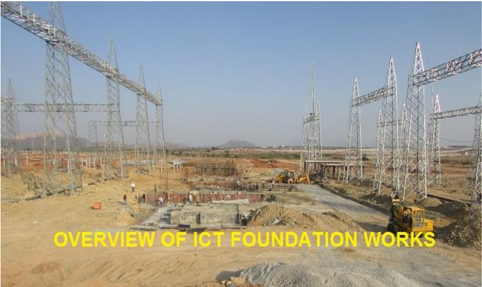
ICT FOUNDATIONS WORKS IN PROGRESS – OVERVIEW AT NP KUNTA 400/220KV SS
