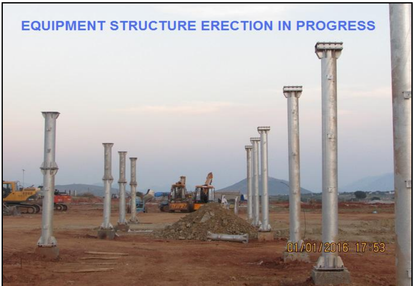
EQUIPMENT STRUCTURES ERECTION IN PROGRESS
