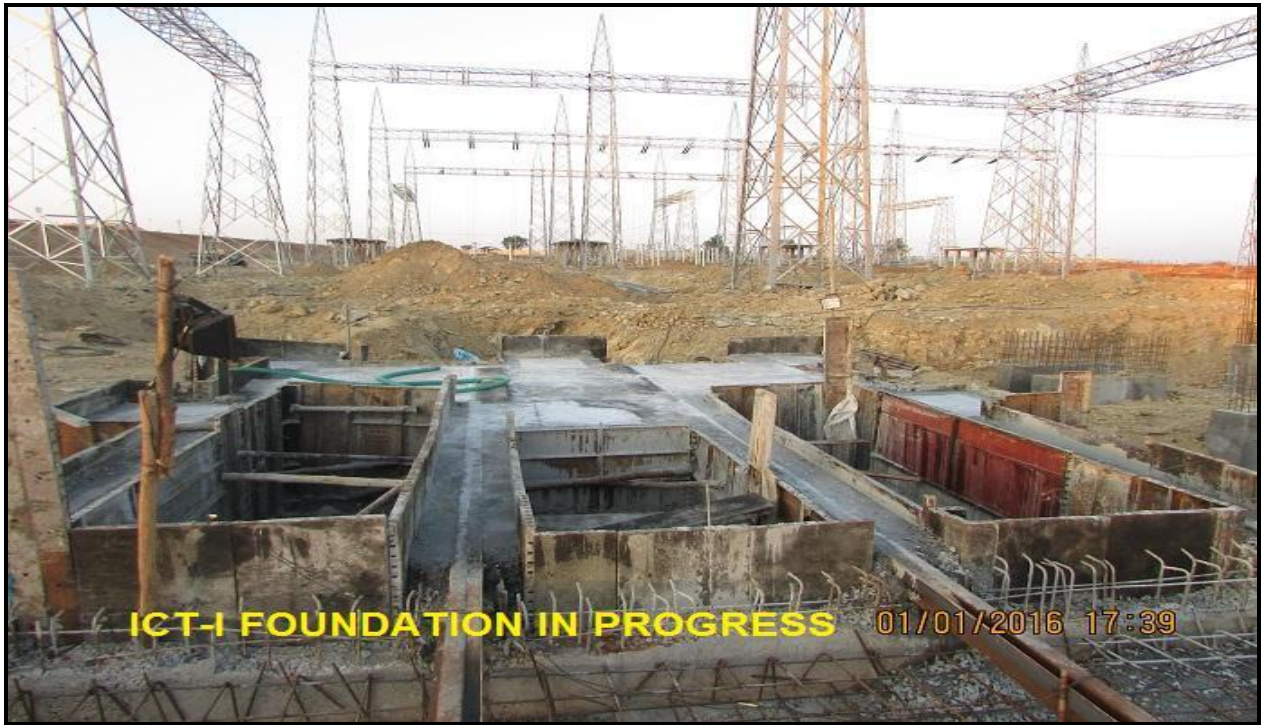
ICT-I FOUNDATION IN PROGRESS
