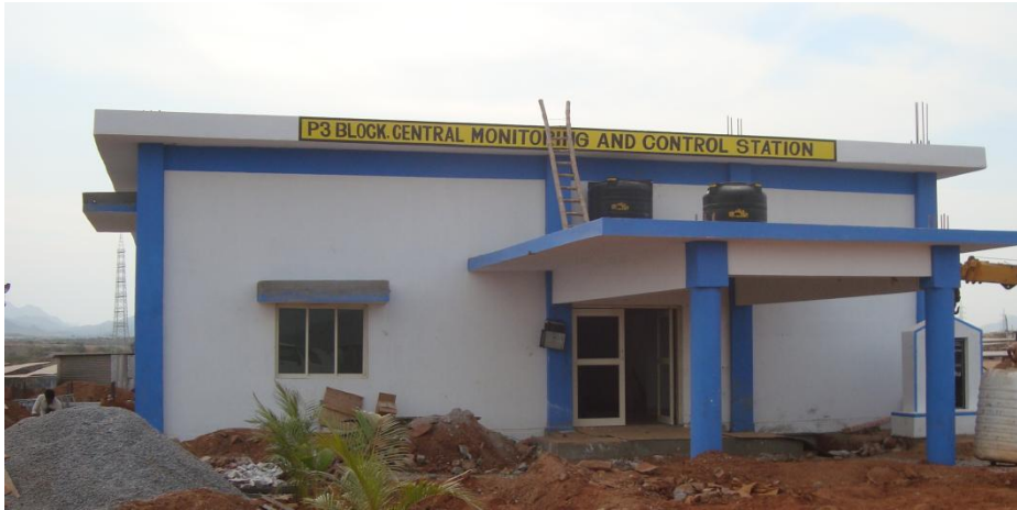
Figure-3: CMCS building of P-3 block (M/s Lanco) as on 29.02.2016
