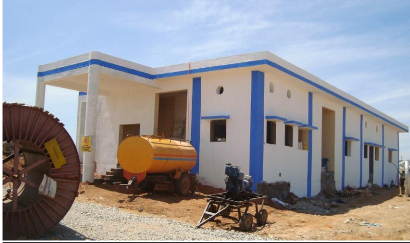
Figure-1: CMCS building of P-2 block (M/s Tata) as on 29.02.2016
